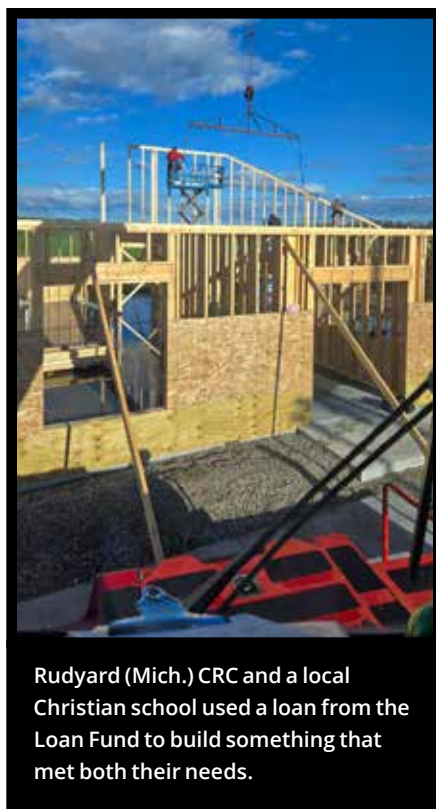
Photo by Mike Ross, general contractor, Whiskey River Inc.
